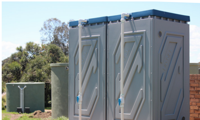
Two bioreactors were added to the existing sewage treatment plant.
