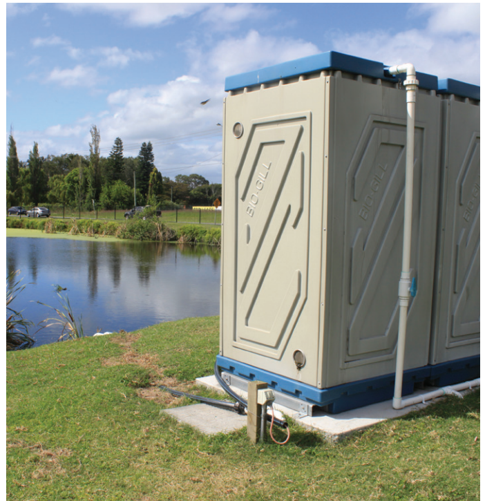
BioGill bioreactors treating wastewater onsite at Tomago.
