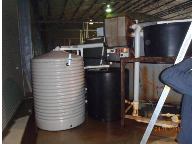
Figure 1 BioGill Unit (white) as part of the recirculating aquaculture system at PSFI Hatchery
